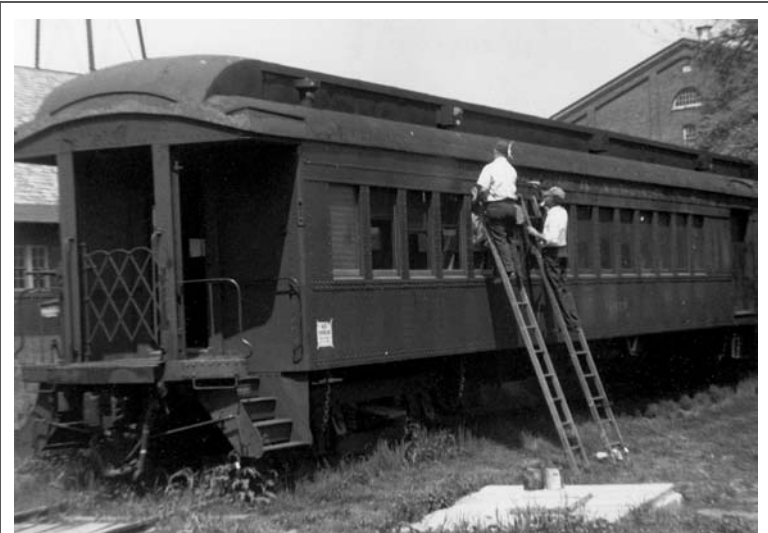
Combine 410 undergoes restoration by founder Thomas C. Marshall, Jr. and charter member Pete Small in Yorklyn. The “Lackawanna” livery above the windows is being removed at the Worth Brothers siding at the former Garrett Snuff Mills on May 12, 1962. The coaches are painted a blue with yellow window highlights recognizing both the B&O and the State of Delaware. “Wilmington & Western” will be lettered in yellow is across the top of the windows. Delaware’s state colors are Colonial Blue and Buff and the B&O’s colors are Royal Blue and Gold. Richard Hall photo.
