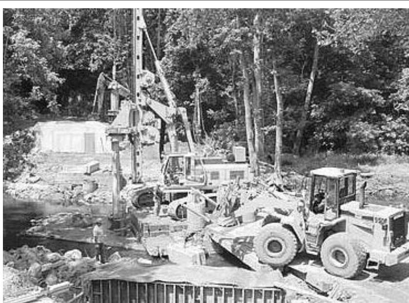
The replacement trestles 6C (Greenbank) and 6G (Brandywine Springs) are designed with 36" concrete and steel piles drilled down to bedrock beneath the Red Clay Creek which support and anchor the concrete islands constructed on the creek bed. With fewer supports (bents) in the creek, there is less opportunity for trees, branches, and other debris to build against the bents and damage the trestle during severe tropical storms and hurricanes occasionally visiting the Red Clay Valley. David Ludlow photo.
