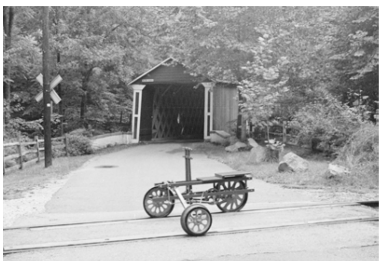
The editor's Sheffield No. 1 Velocipede at Wooddale in September 1992. After the Wilmington & Western Rail Road Company started using the line in 1872, velocipedes would have seen use after 1877 by workers for inspections and maintenance activities. A one-person velocipede was designed to carry a maximum load of 300 pounds. The No. 1 featured machine-cut gearing, ball bearing axles, and concave tread on the two large wheels to “practically eliminate the tendency to leave a wet or frosty rail”. Operating a velocipede is similar to sculling were the rider pushes pedals with their feet while pulling the vertical handle with their hands. The two handle positions serve as a “transmission”. The upper handles allow maximum leverage to get moving and then the operator uses the lower handles to keep moving and thus limit the rocking necessary for their upper body. Robert. E. Wilhelm, Jr. photo.
