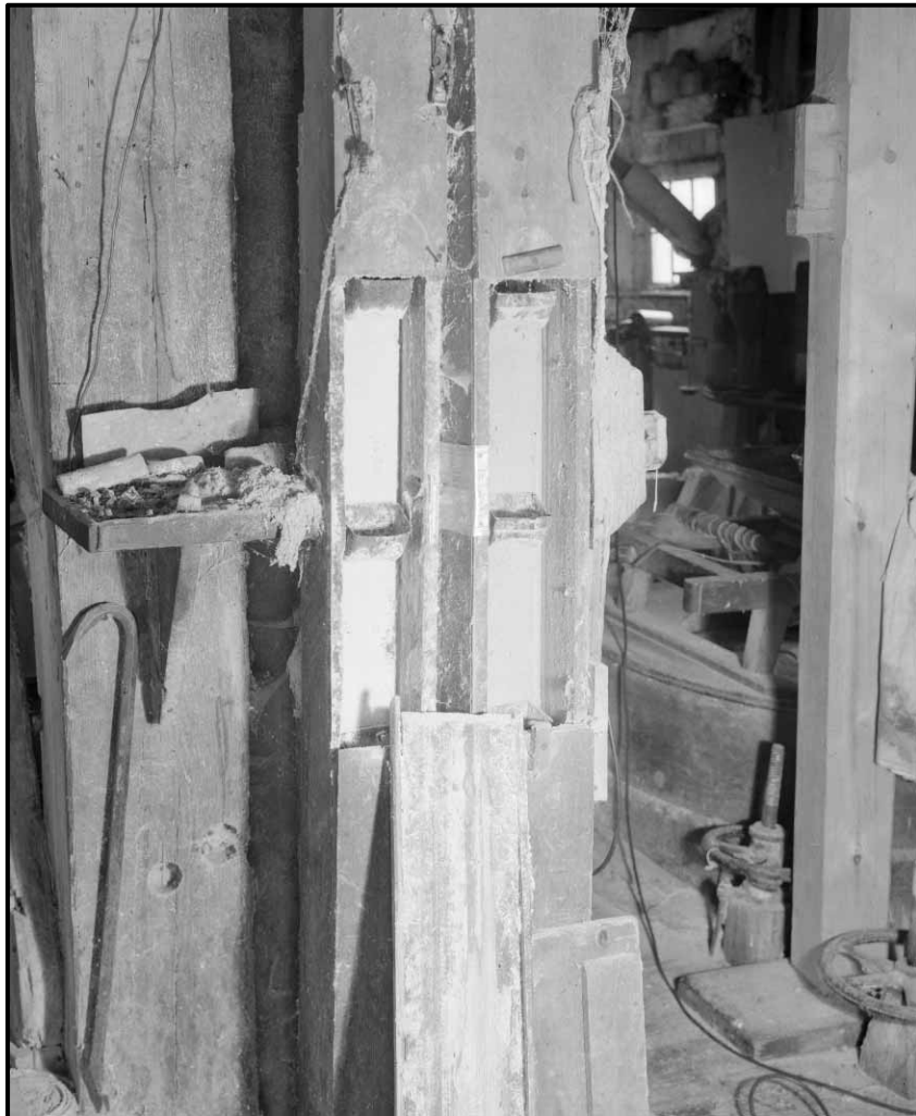
Evans Bucket Ascending Conveyor (access door removed)
