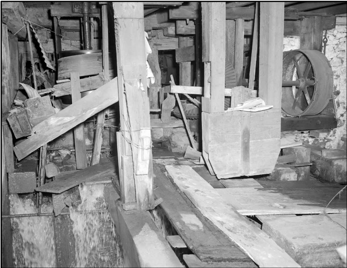
Turbine wheel pit (left, right rear), Evan's bucket elevator (right, foreground)
